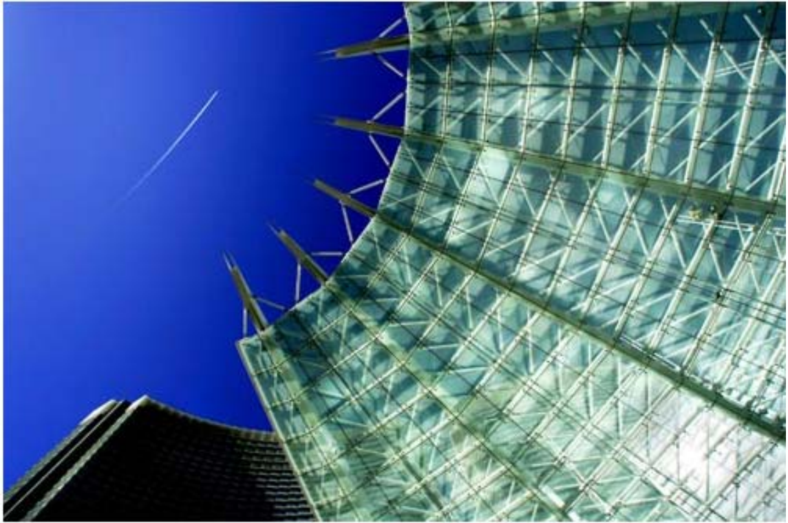
(Ricardo DeAratanha / Los Angeles Times) Canopy over the porte-cochere of Aria Resort & Casino.
